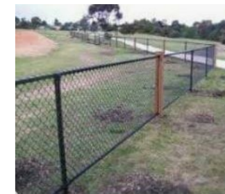
EXAMPLE PHOTO OF MESH FENCE
